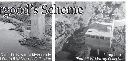
Some water would drive a turbine which coupled to a pump, the pumped water was to be taken across the river in a pipe known as a rising main to a holding dam. From here via open water races to irrigate the land between the mouth of the Kawarau Gorge to Cromwell and as far as Lowburn.
